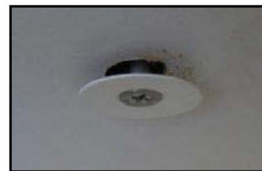
EXAMPLE OF LOOSENED FASTENER ELEMENT
