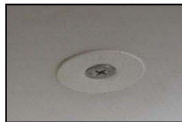
EXAMPLE OF CORRECTLY INSTALLED FASTENER ELEMENT
