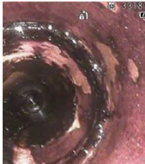
BROWN SURFACE VARNISH EXAMPLE (ACCEPTABLE CONDITION)
