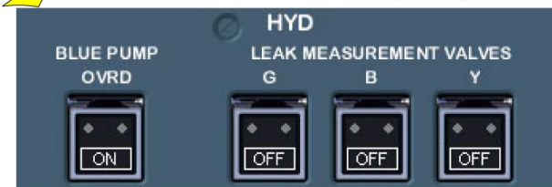
MAINTENANCE PANEL (50VU)
